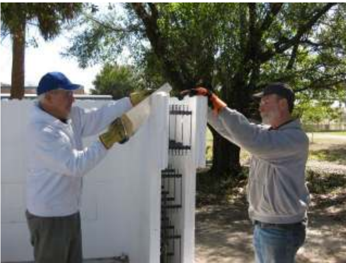
Tom and Marty building a wall
